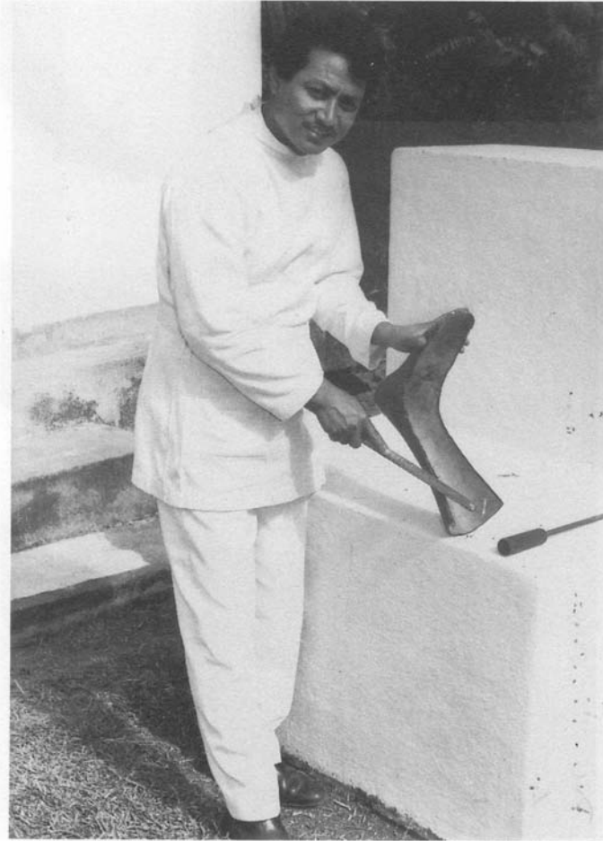
Figure 10. The cut edges are smoothed while the PVC is still warm.
