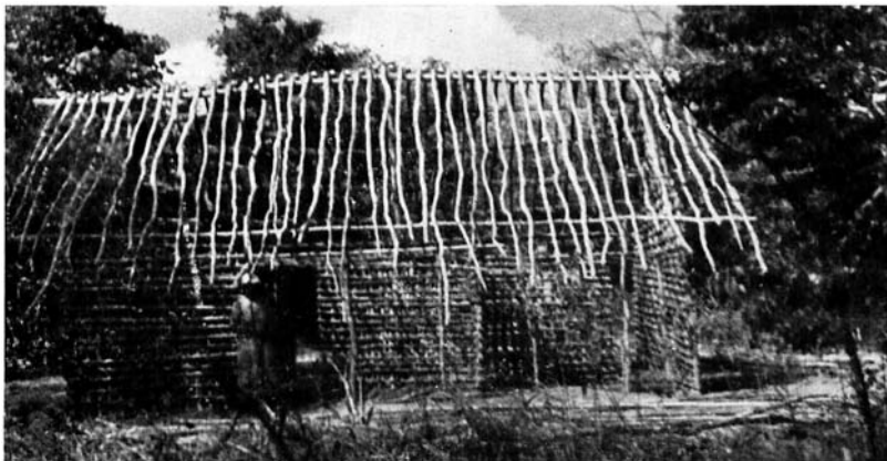
The simple hut of self-supporting lepers in S. Tanganyika made of branches tied together with bark rope. The grass thatch of the roof and mud plaster of the walls have still to be added.
