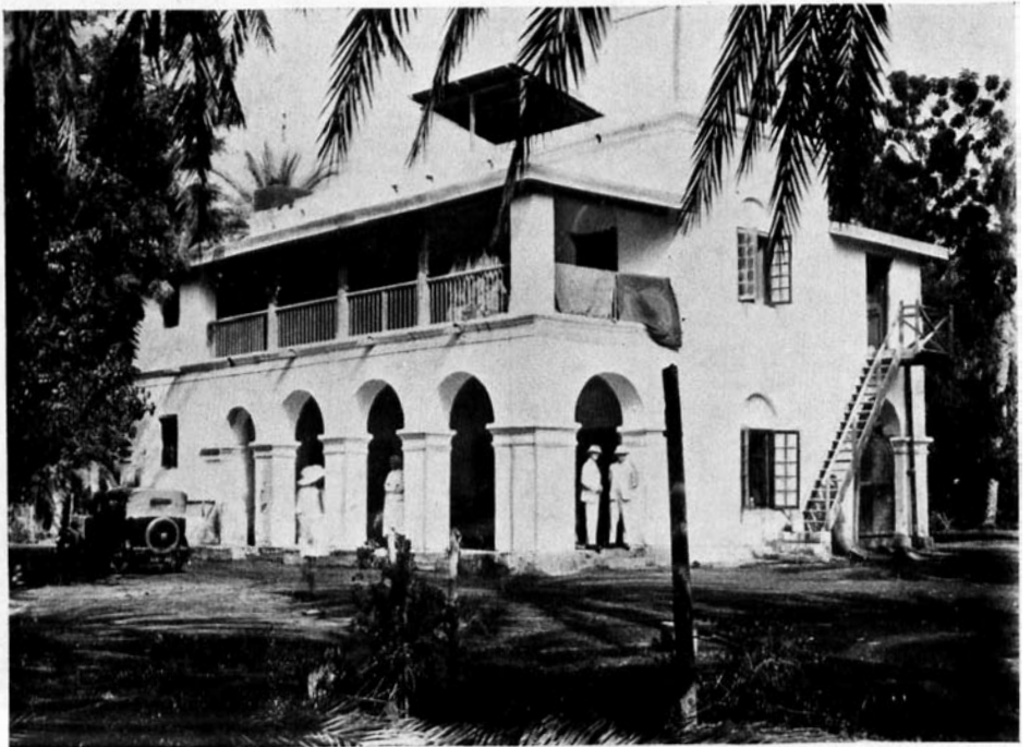
General View of the Hospital Building.
